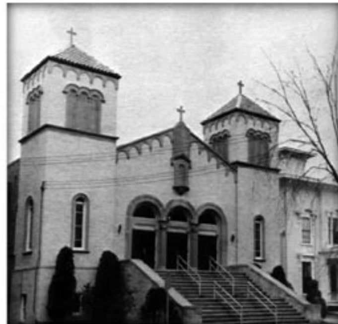
Above: Saint Barbara Greek Orthodox Church 56 Dwight Street, New Haven
